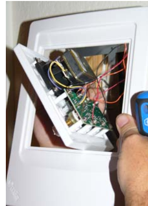
Figure 8 - Placing Room Station in
